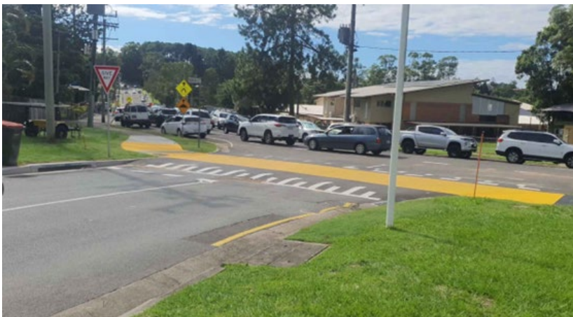
Figure 1.2 – Example of a raised priority crossing for a shared pathway, Bli Bli, Qld
