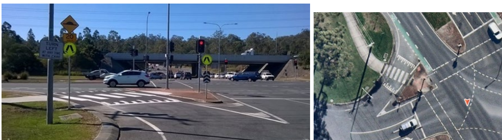
Figure 5.3(a) – Raised crossing with ramps perpendicular to direction of vehicle travel on slip lane, Entertainment Road, Oxenford, Qld
