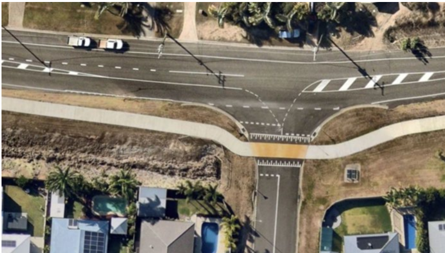
Figure 3(d) – Urban channelised right turn on approach to a raised priority crossing provides a safe place for vehicles to slow down and store whilst checking for vehicles and path users (Winton Way and Coronation Drive, Tannum Sands)
