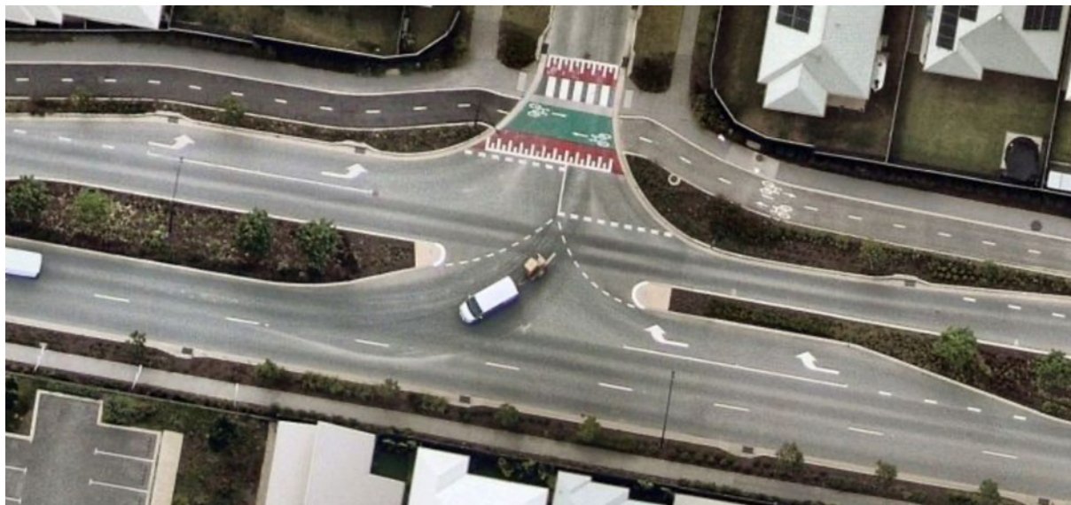
Figure 3(e) – Auxiliary and Channelised turn lanes at approaches to separated pedestrian and cyclist crossing provide (Banaya Ave and Terrance Ave, Nirimba)
