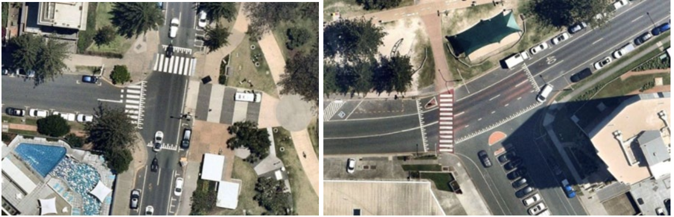
Figure 3(c) – Left: Raised intersection with priority crossings (Northcliffe Tce, Surfers Paradise). Right: Ramps designed perpendicular to vehicular path of travel (Ward St, Tweed Heads)
