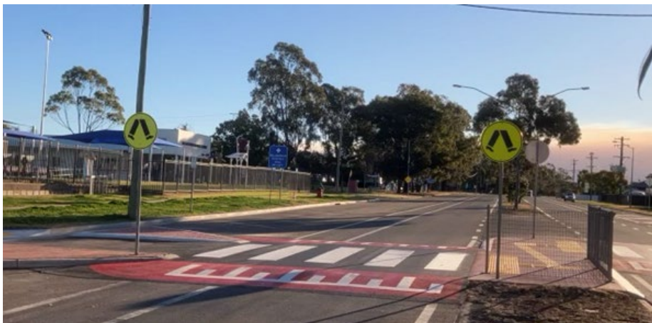
Figure 4.2(b): Raised pedestrian crossing incorporating red pavement treatments on ramps. Red pavement should not be provided beneath zebra crossing markings. Gore Hwy, Milmerran
