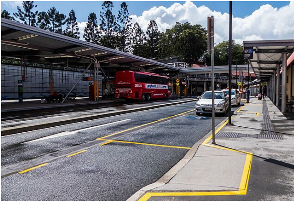
Figure 40 Roma Street Station passenger loading zone
