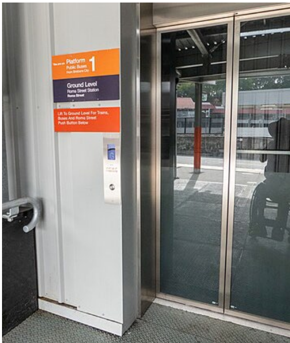
Figure 197 Braille and tactile wayfinding sign at lift, Roma Street bus station
