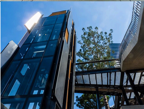
Figure 172 Lift car, North Quay ferry terminal
