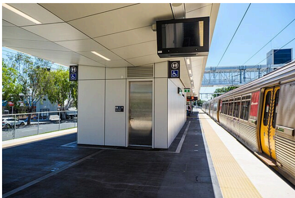
Figure 188 Toilet signage, Yeronga rail station
