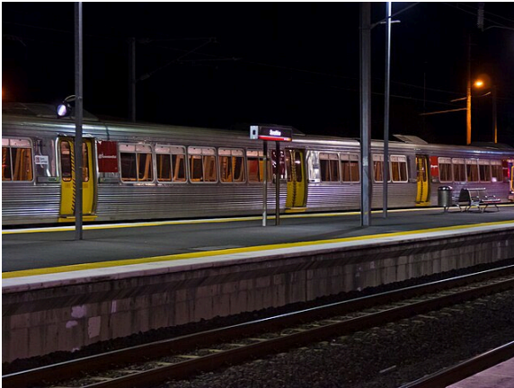
Figure 140 Lighting at Sunshine rail station, Geebung
