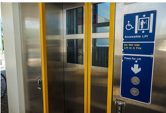
Figure 167 Lift signage, Fairfield rail station
