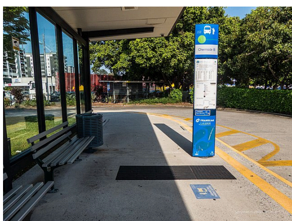
Figure 193 Next service information, Chermide bus interchange
