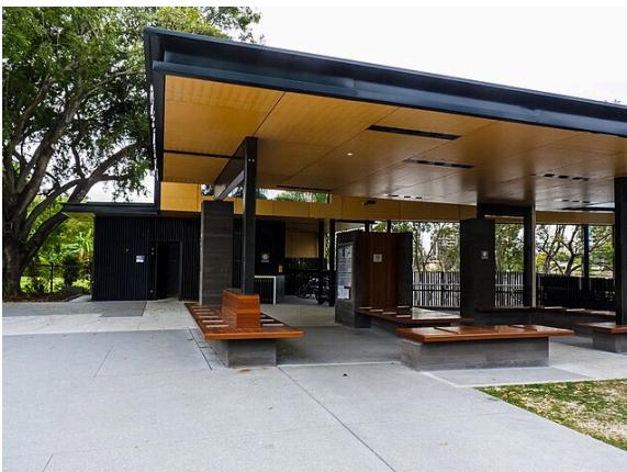
Figure 97 Terminal amenities, West End ferry terminal
