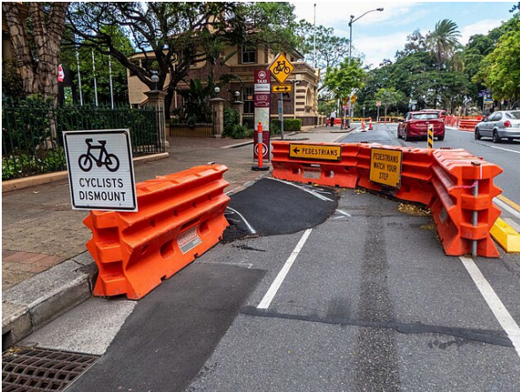
Figure 21 Temporary kerb ramp, Edward Street, Brisbane
