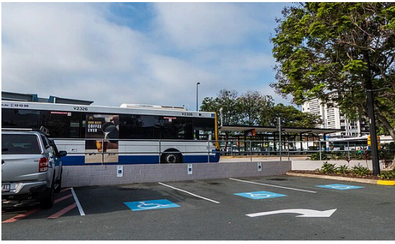
Figure 70 Accessible parking, Chermside bus interchange
