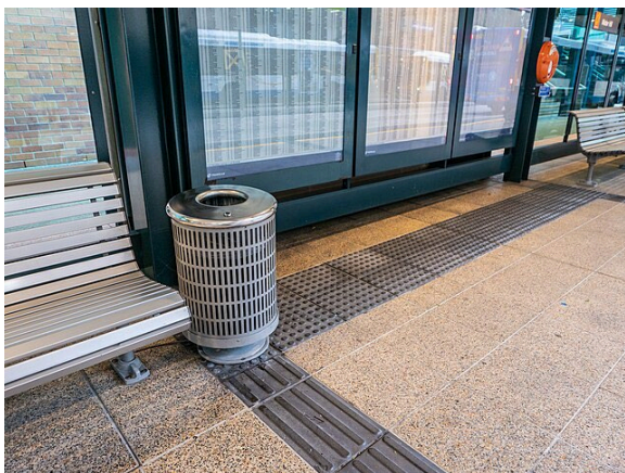
Figure 210 TGSI, Mater Hill bus station
