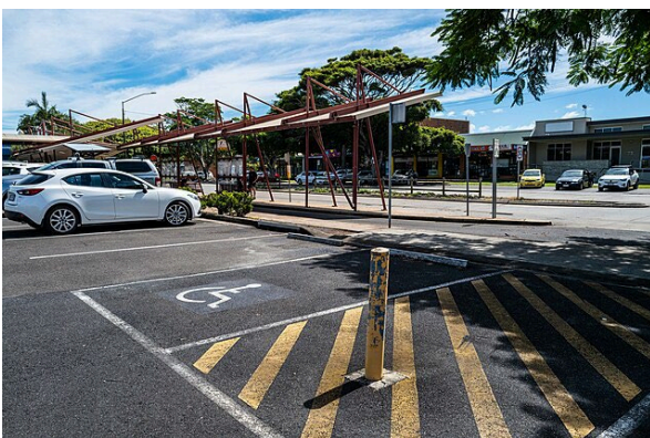
Figure 43 Tamar Street accessible parking, Ballina, NSW
