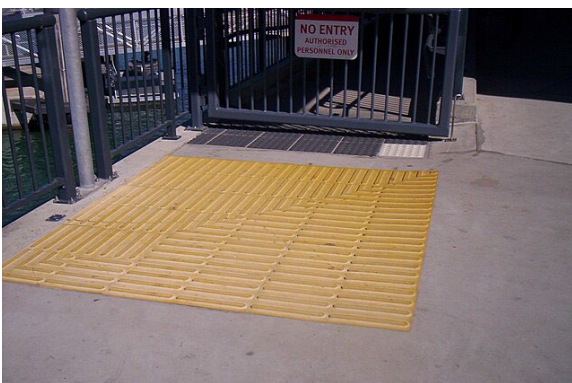
Figure 219 TGSI, Nelly Bay ferry terminal, Magnetic Island
