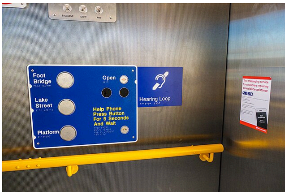
Figure 154 Lift help phone, Yeronga rail station
