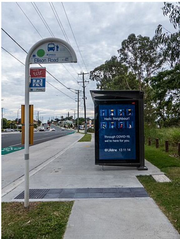
Figure 232 Bus stop TGSIs, Murphy Road, Chermside
