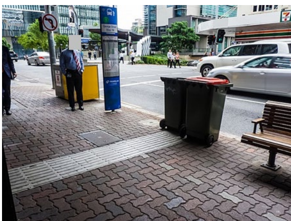
Figure 211 TGSI, George Street, Brisbane
