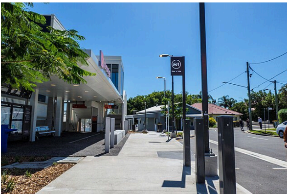
Figure 23 Passenger loading zone, Yeronga Rail Station
