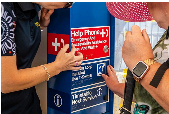
Figure 156 Platform help phone, Cultural Centre bus station
