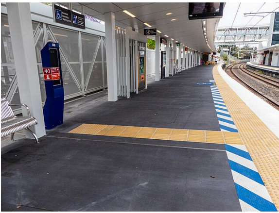
Figure 208 TGSI, Fairfield rail station
