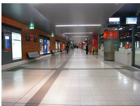
Figure 138 Lighting at King George Square bus station, Brisbane
