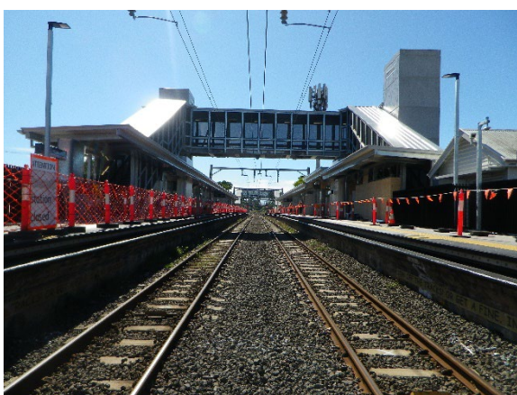
Figure 37 Royal Parade level crossing at Banyo Station 2025.
