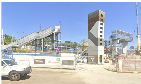
Figure 174 Lift and stairs during construction, Morningside station, 2024
