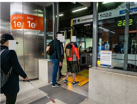
Figure 235 TGSI, King George Square bus station, Brisbane
