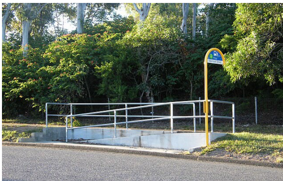
Figure 116 Footpath at higher grade than roadway, Ellison Road, Geebung
