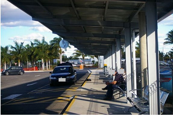
Figure 51 Passenger loading zone, Rockhampton Airport.
