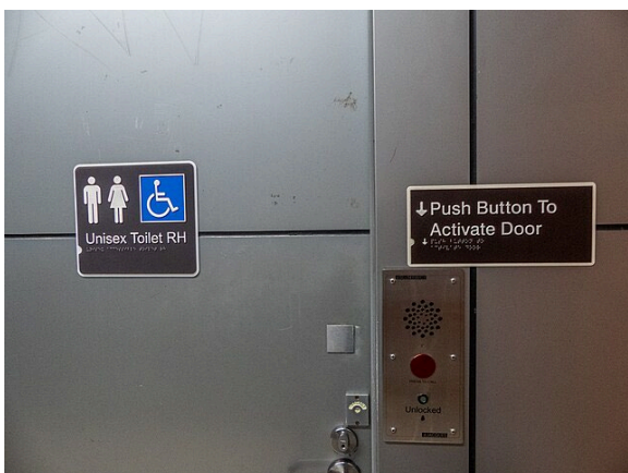
Figure 191 Toilet intercom, King George Square bus station
