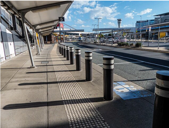
Figure 234 TGSI, Brisbane Domestic Terminal, Brisbane Airport
