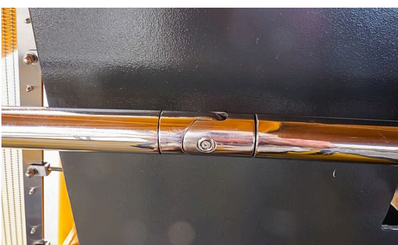
Figure 99 Handrail joint, QUT Gardens Point ferry terminal
