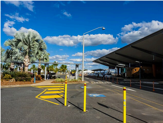
Figure 67 Accessible parking, Rockhampton airport
