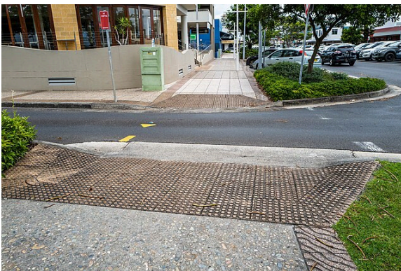
Figure 217 TGSI Ballina, New South Wales
