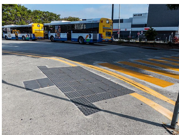
Figure 221 TGSI, Chermside bus station
