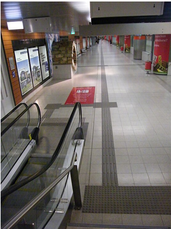
Figure 202 Directional TGSi, King George Square bus station
