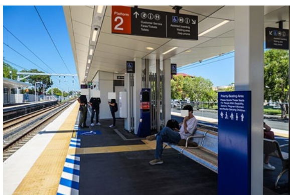
Figure 230 Platform TGSI, Yeronga rail station
