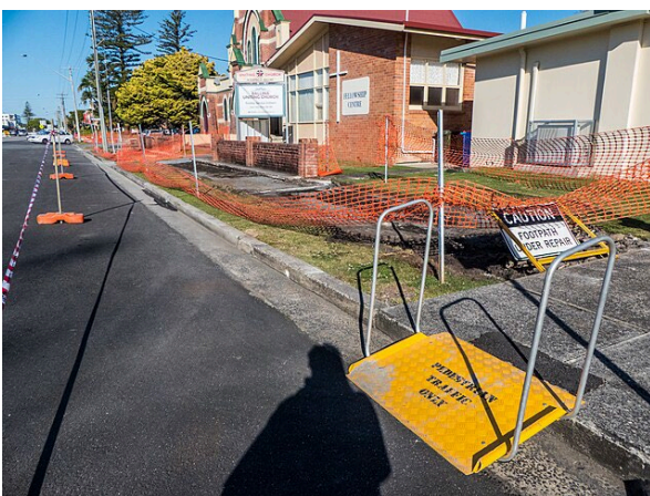
Figure 20 Temporary kerb ramp, Cherry Street, Ballina, NSW
