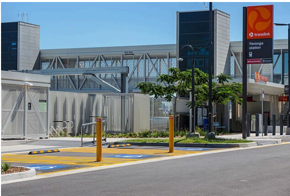
Figure 60 Accessible parking signage, Lake Street, Yeronga station
