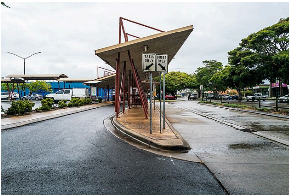
Figure 42 Tamar Street bus interchange and taxi zones, Ballina, NSW
