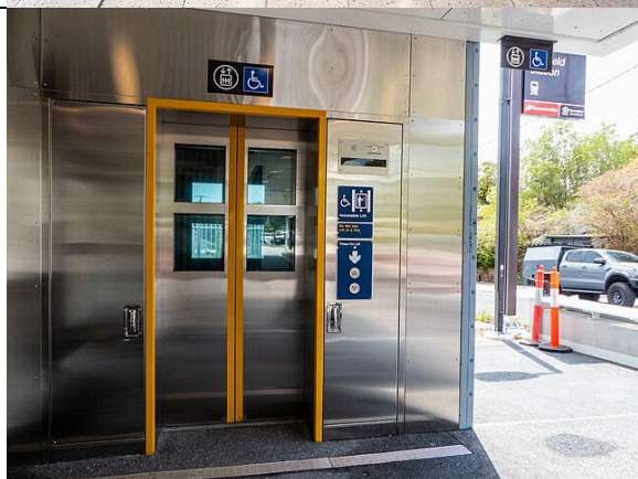
Figure 164 Lift doors, Yeronga rail station
