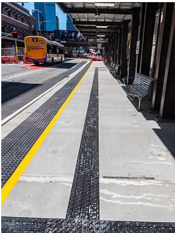
Figure 203 TGSIs, Cultural centre bus station
