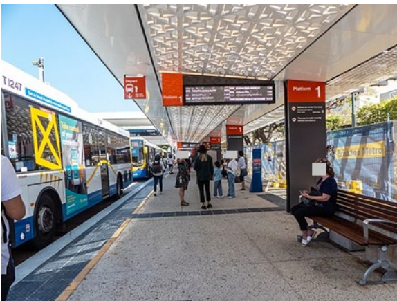
Figure 82 Station amenities, Cultural Centre bus station Good practice: Boarding points, information displays, TGSIs, seats and signs are covered by DSAPT-2002, Cultural Centre bus station.
