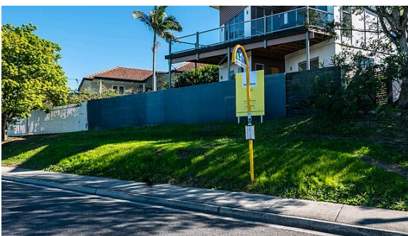
Figure 115 Bus stop located with steep crossfall, Edinburgh Castle Road, Wavell Heights
