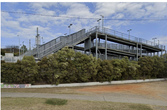
Figure 173 Access ramp, Morningside rail station, 2008
