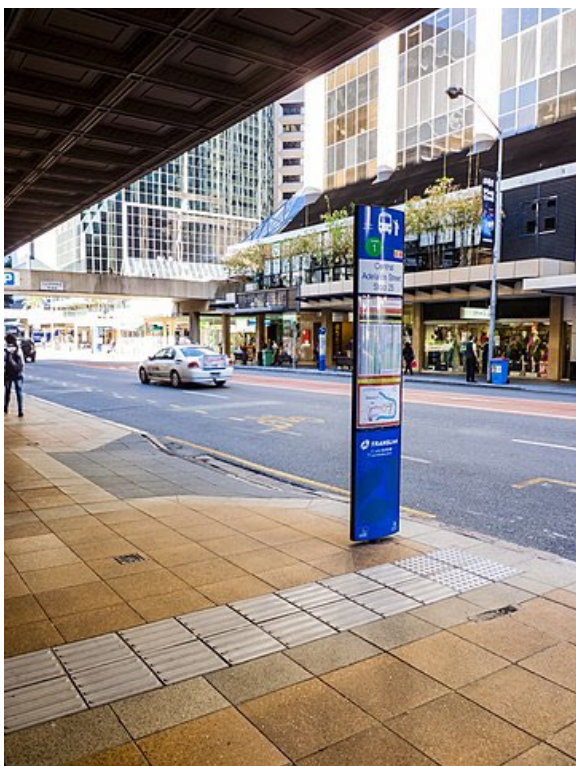
Figure 233 Bus stop TGSIs, Adelaide Street, Brisbane
