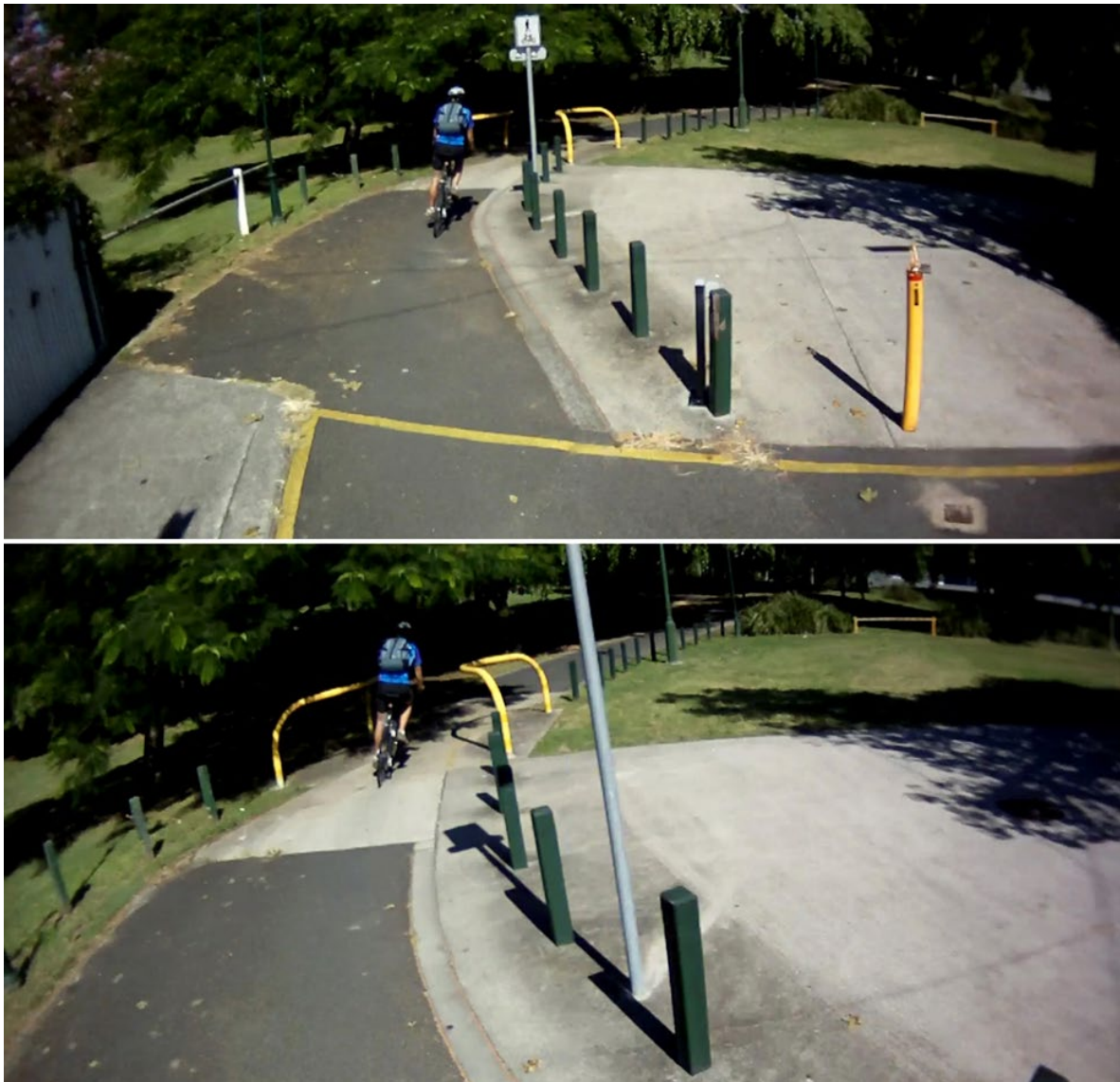
Figure C.21 – Illustration of people riding bikes ‘lean into’ corner turns, and the hazardous positioning of this terminal barrier
