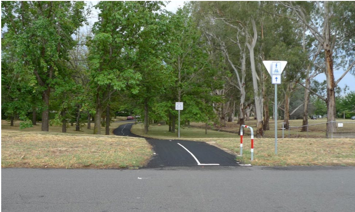
Figure C.1 – Path with minimal termination treatment
