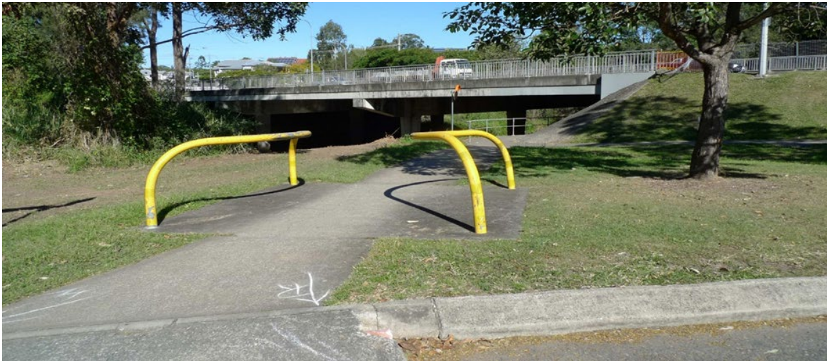
Figure C.3 – Redundant path terminal barrier
