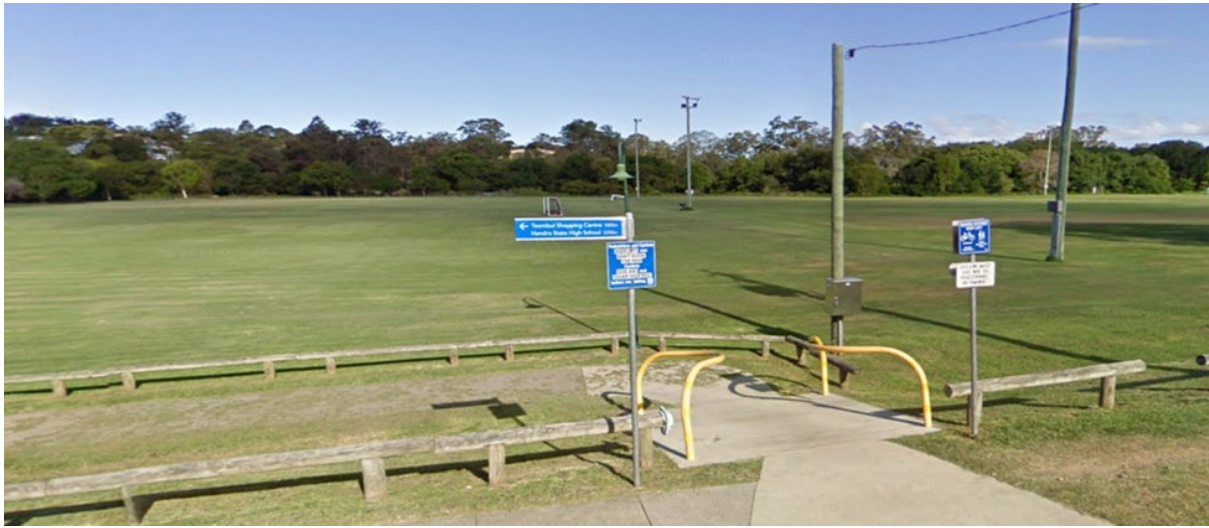
Figure C.6 – Hazardous positioning of a path terminal barrier
