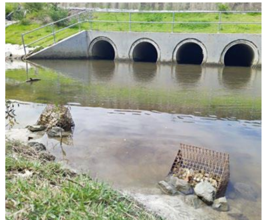
Figure 12: Installed robust oyster baskets and quilted oyster doonas to enhance marine biodiversity. Source: © State of Queensland
